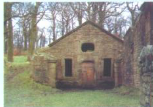
3. Hollinshead Hall: haunted Well House
