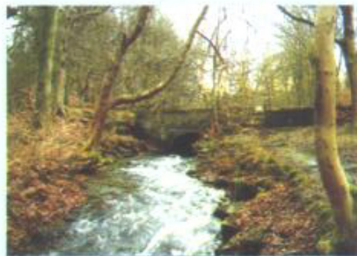
3. Bridge over the River Roddlesworth
