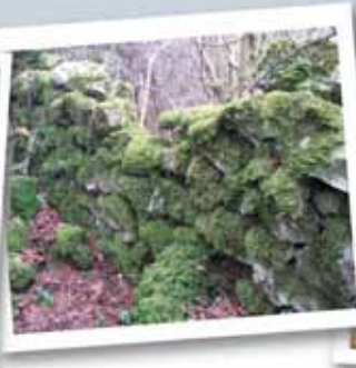
Historic boundary wall
